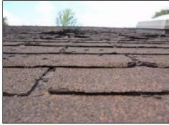
DETERIORATING SHINGLES
