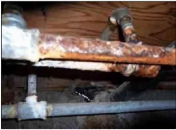
RUSTED PIPES
