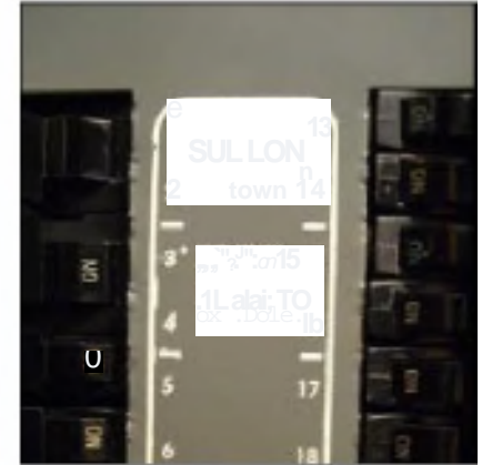
The above photos show Federal Pacific/Stab-Lok electrical panes. Both the white or black (mapping) box or brown paper labels are clear indications that the panel is a Federal Pacific! Stab-Lok electrical panel.
