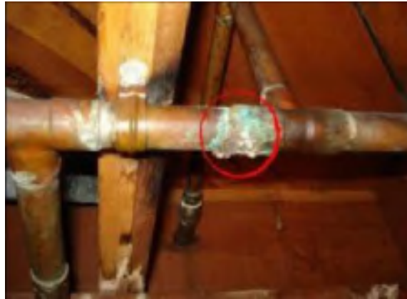
CORRODED PIPES
