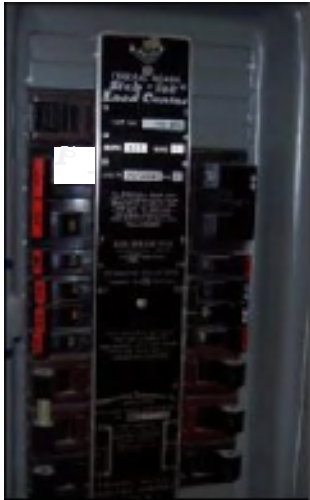
The above photos show Federal Pacific/Stab-Lok electrical panes. Both the white or black (mapping) box or brown paper labels are clear indications that the panel is a Federal Pacific! Stab-Lok electrical panel.
