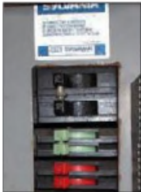
The above photos show Zinsco/Sylvania electrical panels. They often have a branding sticker, and another clear indicator is that the breakers are typically colored light blue, light green and red. NOTE: Although a photo of the Challenger electrical panels is not included above, these panels are also considered Ineligible as detailed on page 13.
