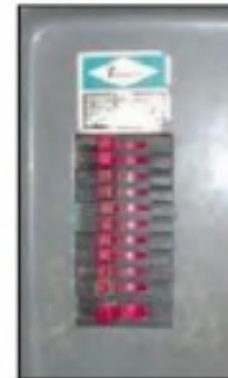
The above photos show Zinsco/Sylvania electrical panels. They often have a branding sticker, and another clear indicator is that the breakers are typically colored light blue, light green and red. NOTE: Although a photo of the Challenger electrical panels is not included above, these panels are also considered Ineligible as detailed on page 13.
