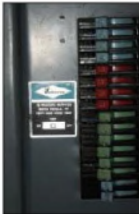
The above photos show Zinsco/Sylvania electrical panels. They often have a branding sticker, and another clear indicator is that the breakers are typically colored light blue, light green and red. NOTE: Although a photo of the Challenger electrical panels is not included above, these panels are also considered Ineligible as detailed on page 13.
