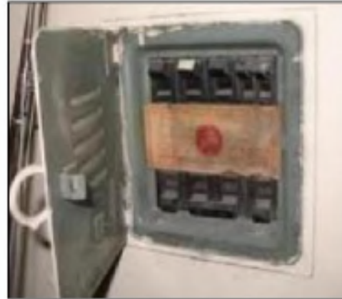
The above photos show Federal Pacific/Stab-Lok electrical panes. Both the white or black (mapping) box or brown paper labels are clear indications that the panel is a Federal Pacific! Stab-Lok electrical panel.
