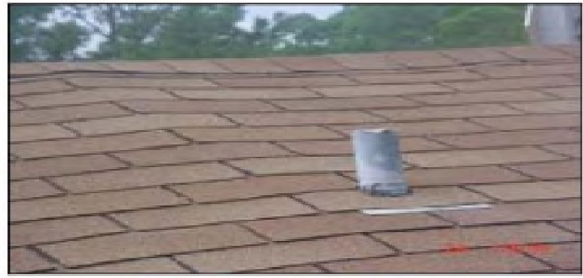
WARPED/ WAVY SHINGLES
