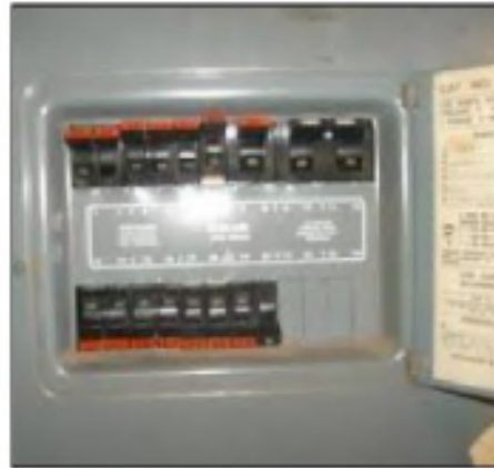
The above photos show Federal Pacific/Stab-Lok electrical panes. Both the white or black (mapping) box or brown paper labels are clear indications that the panel is a Federal Pacific! Stab-Lok electrical panel.
