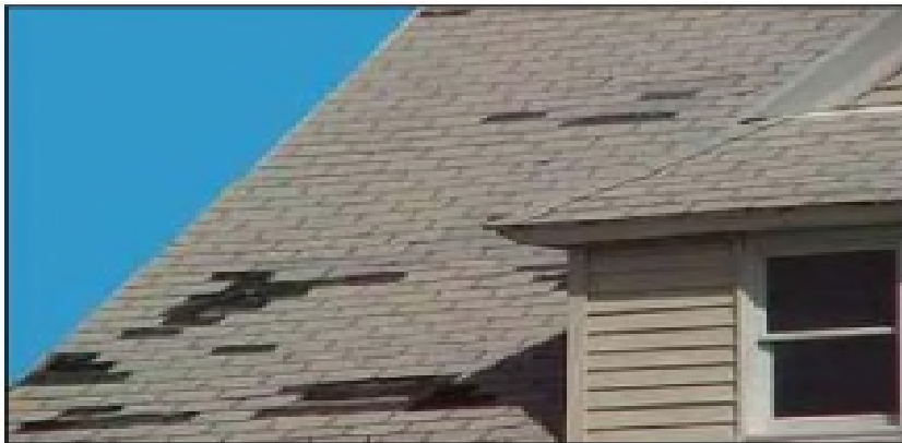
MISSING SHINGLES
